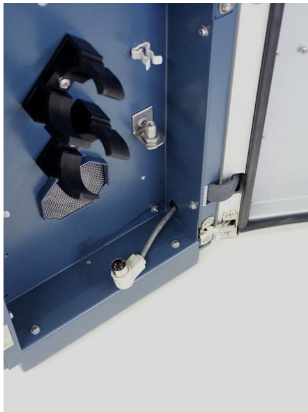
Figure 6. Installation of valve-to-module cable inside DECADE II.
